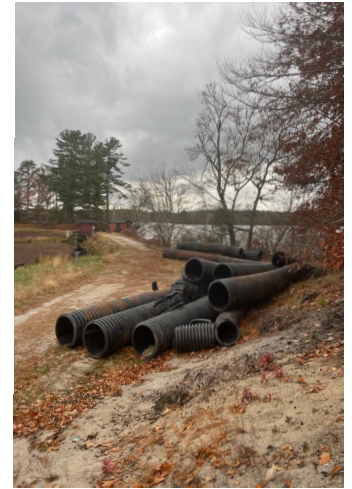
Removed Pipes at Halfway Pond
