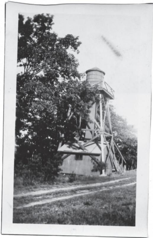
***Back in the early 20th century, families had a steam driven pump at the pond which pumped water up to their water towers. You started the pump, filled the tower and shut off the pump. Gravity served the house fixtures till the tower ran dry again.***
